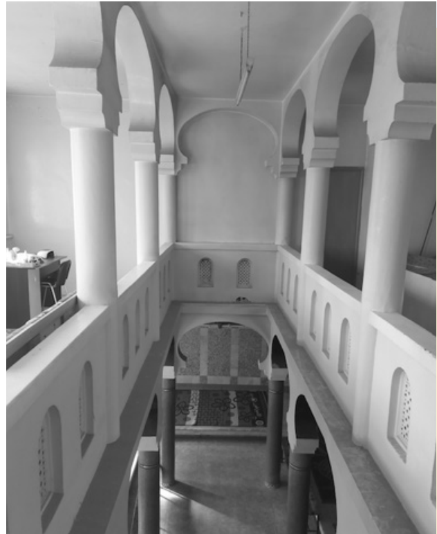
Figure 4 Top view of central patio Source: Author, 2023.
