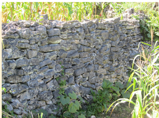
Plate 1 A paril (stone wall structure) built to collect eroded soil. Photo: Zona Amper, April, 2015
